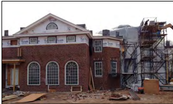
New House Under Construction
